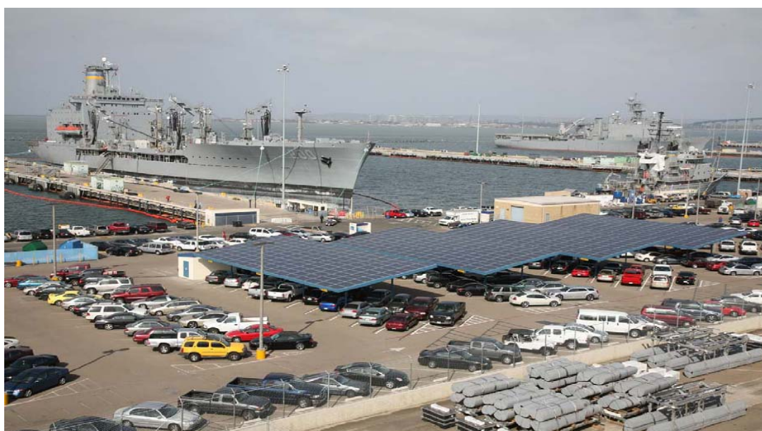
NAVAC Southwest Solar Carport des San Diego Naval Bases
