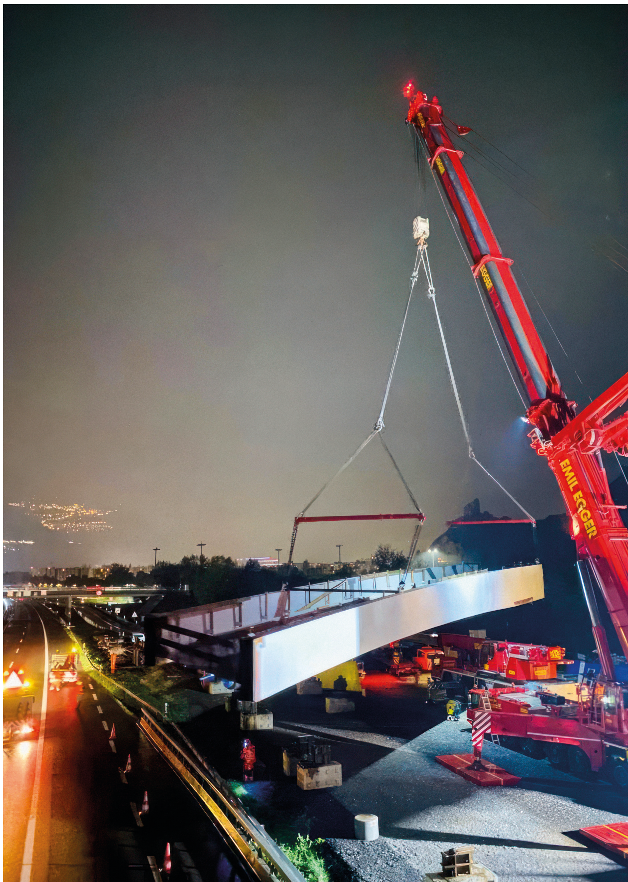
Passerelle A9 de nuit © Alexandre Schmid.
