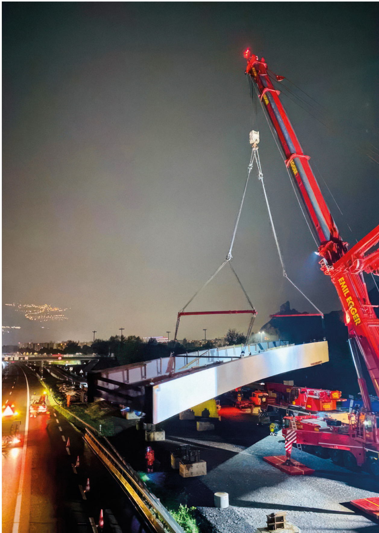
Passerelle A9 de nuit © Alexandre Schmid.
