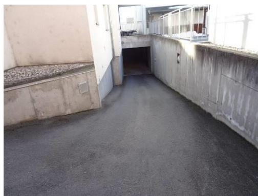
Descente garage souterrain
